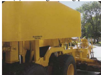
(c) Adding asphalt emulsion
