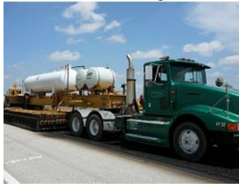
(c) Heating underlying pavement
