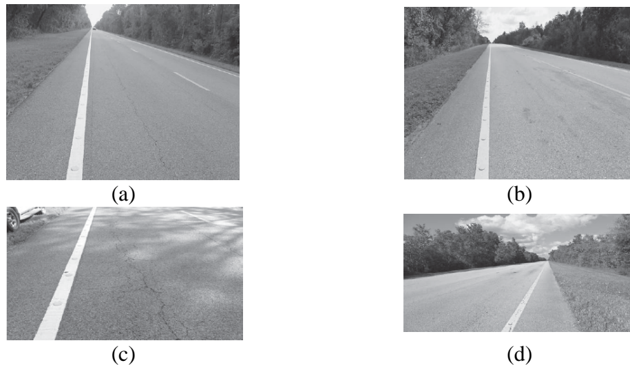
Figure 2-15 a) Average condition of control section (8 years old) b) Average condition of HIR section (8 years old) c) Distressed areas in control section (8 years old) d) Distressed areas in HIR section (8 years old)[57]
