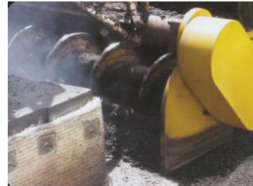
(b) Removing top layer
