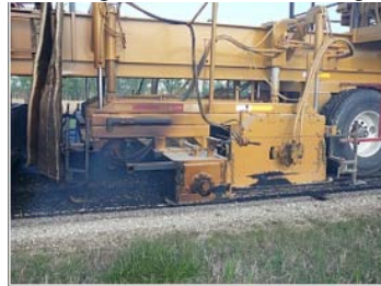
(d) Milling and heating the surface with
