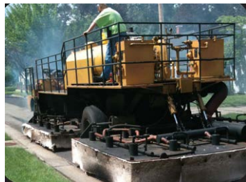
(a) Heating existing pavement
